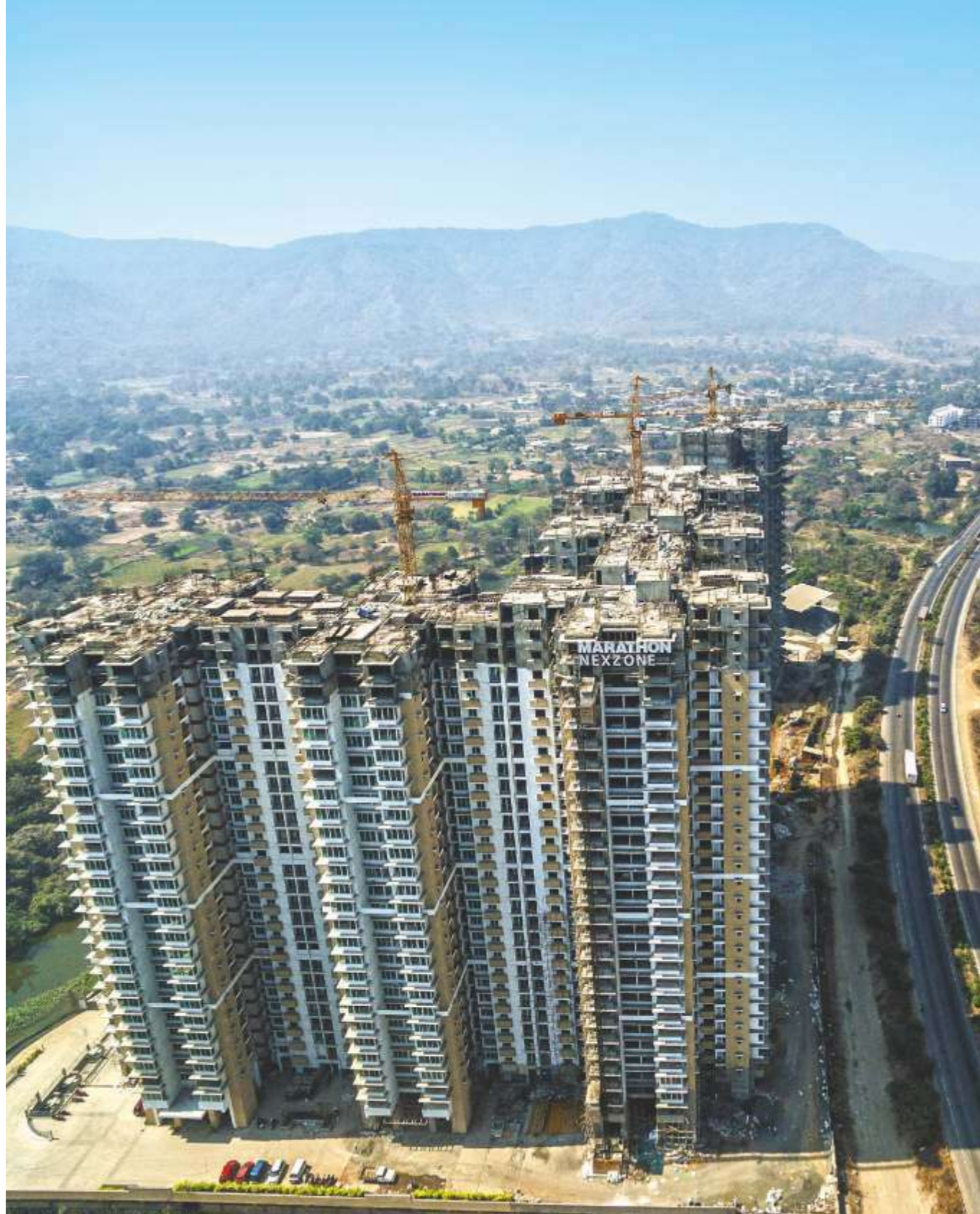
Actual Image - Construction status at Marathon Nexzone
