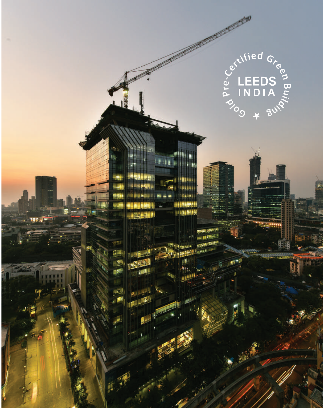
Actual Image - Elevation Construction Status | 27th Slab WIP
